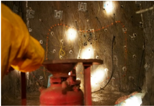
Rock face ready to be blown to bits.
